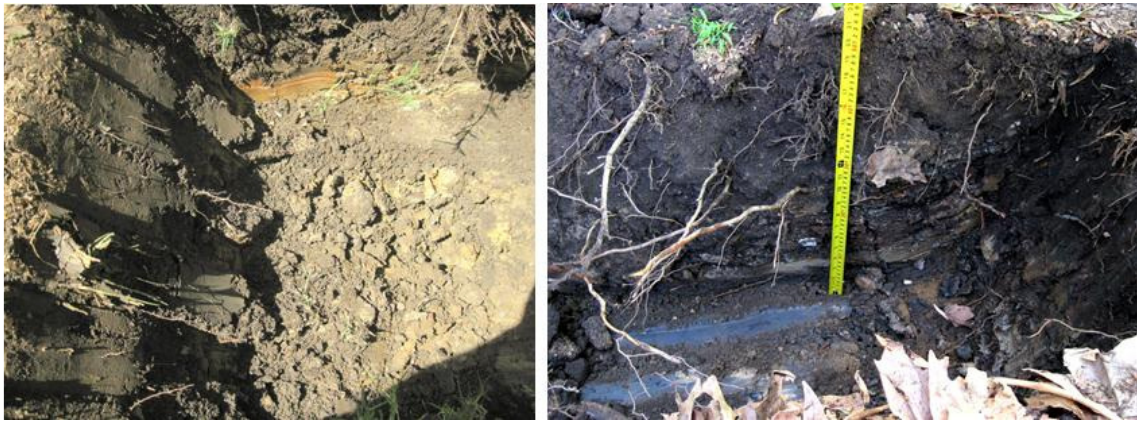
Figure 4.4 – Visual inspection of the opened trenches shows that except for the initial few centimetres of dry top soil the dominant material was clay.
