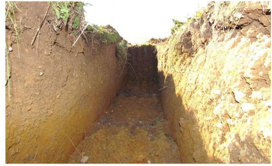
(b) Final trench
